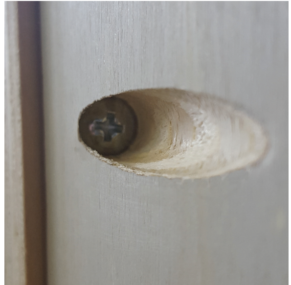
Pocket-screw joinery construction method
